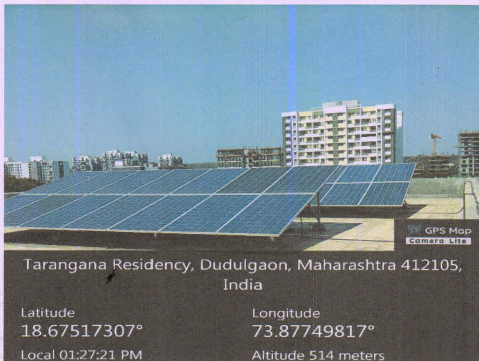
Photograph of 10 kWp Roof Top Solar PV Plant:
